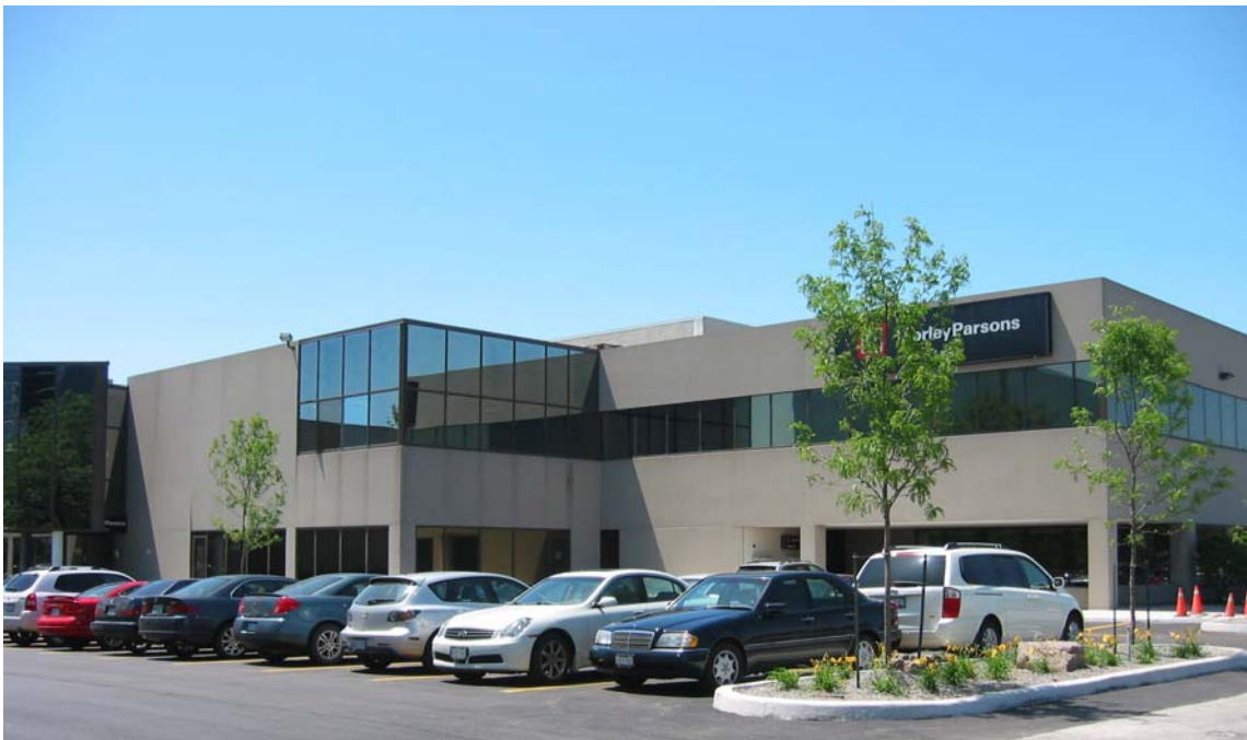
2645 Skymark Avenue, Mississauga
