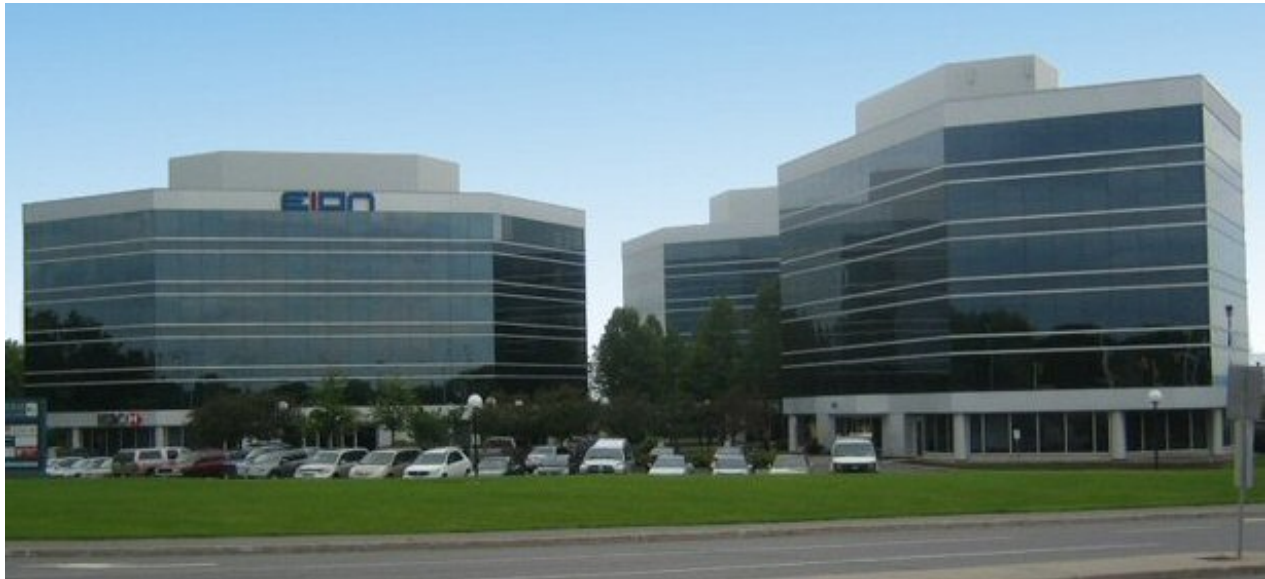
Gateway Office Park, Ottawa
